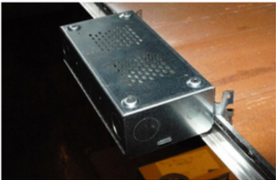
Fig. 49 Mounted to T-Bar using the integral T-Wings
