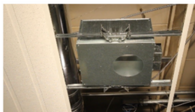
Fig. 70 Downlight suspension from T-bar
