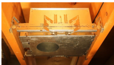
Fig. 69 Downlight suspension from wooden joists
