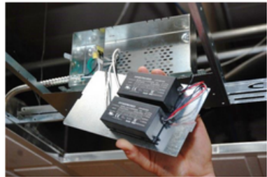
Fig. 48 Mounted to plaster frame with driver installed to cover
